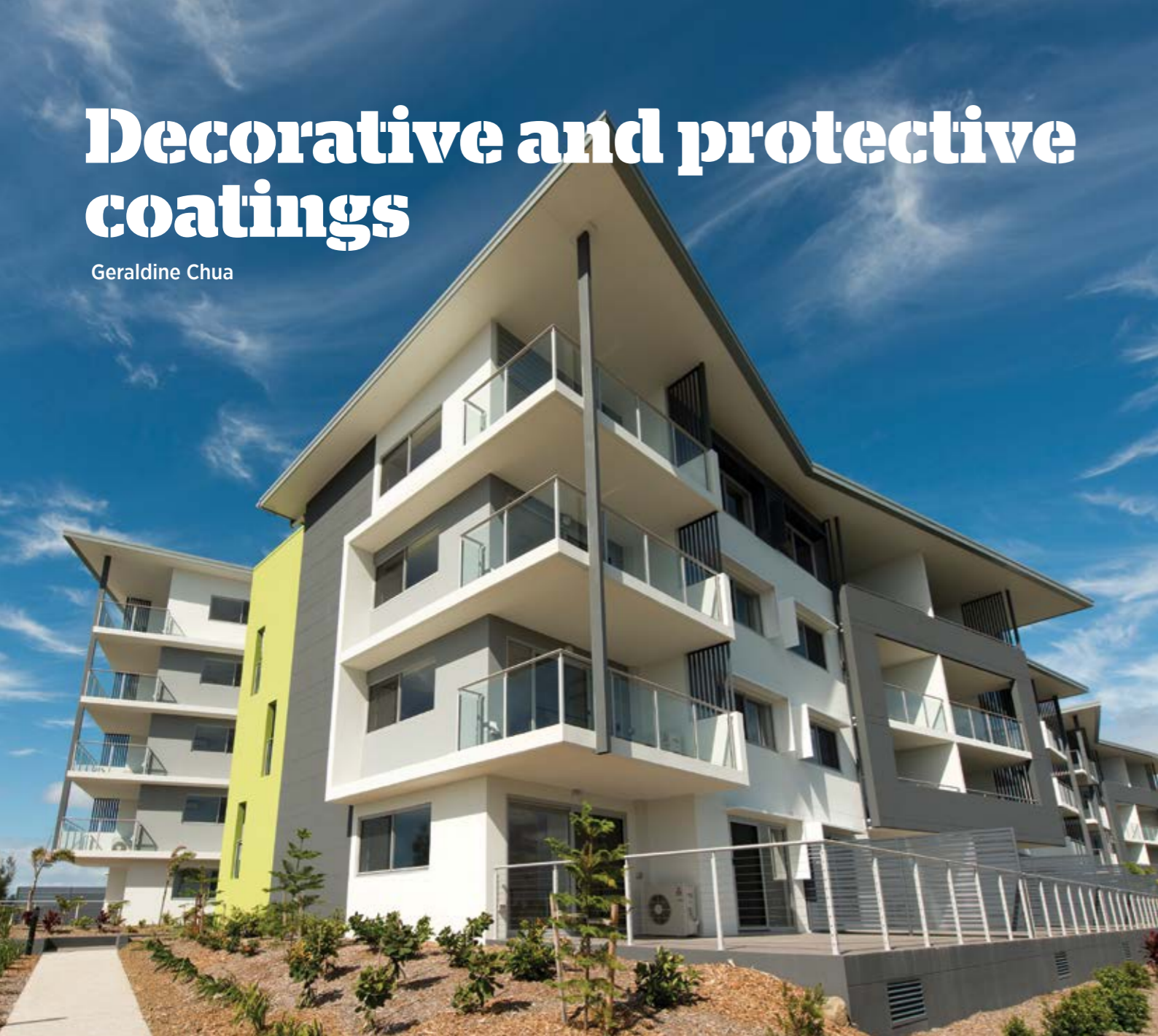
Acrylic texture course was used on the Saltwater Complex at Birtinya, and overcoated with two coats of ROCKCOTE Armour. Image courtesy of ROCKCOTE
